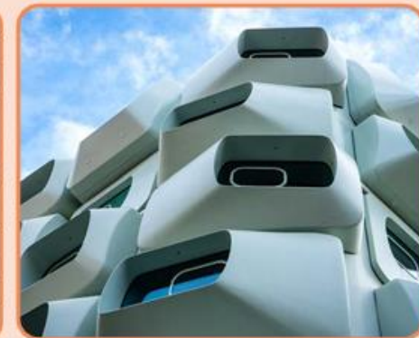
'Argos' building, Austria:
